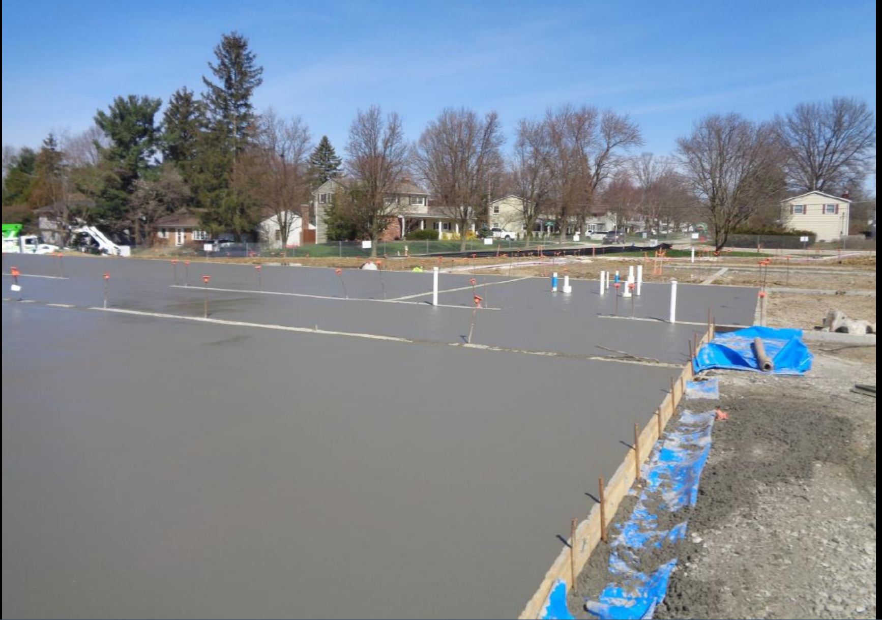
Worthingway Slab Completion
