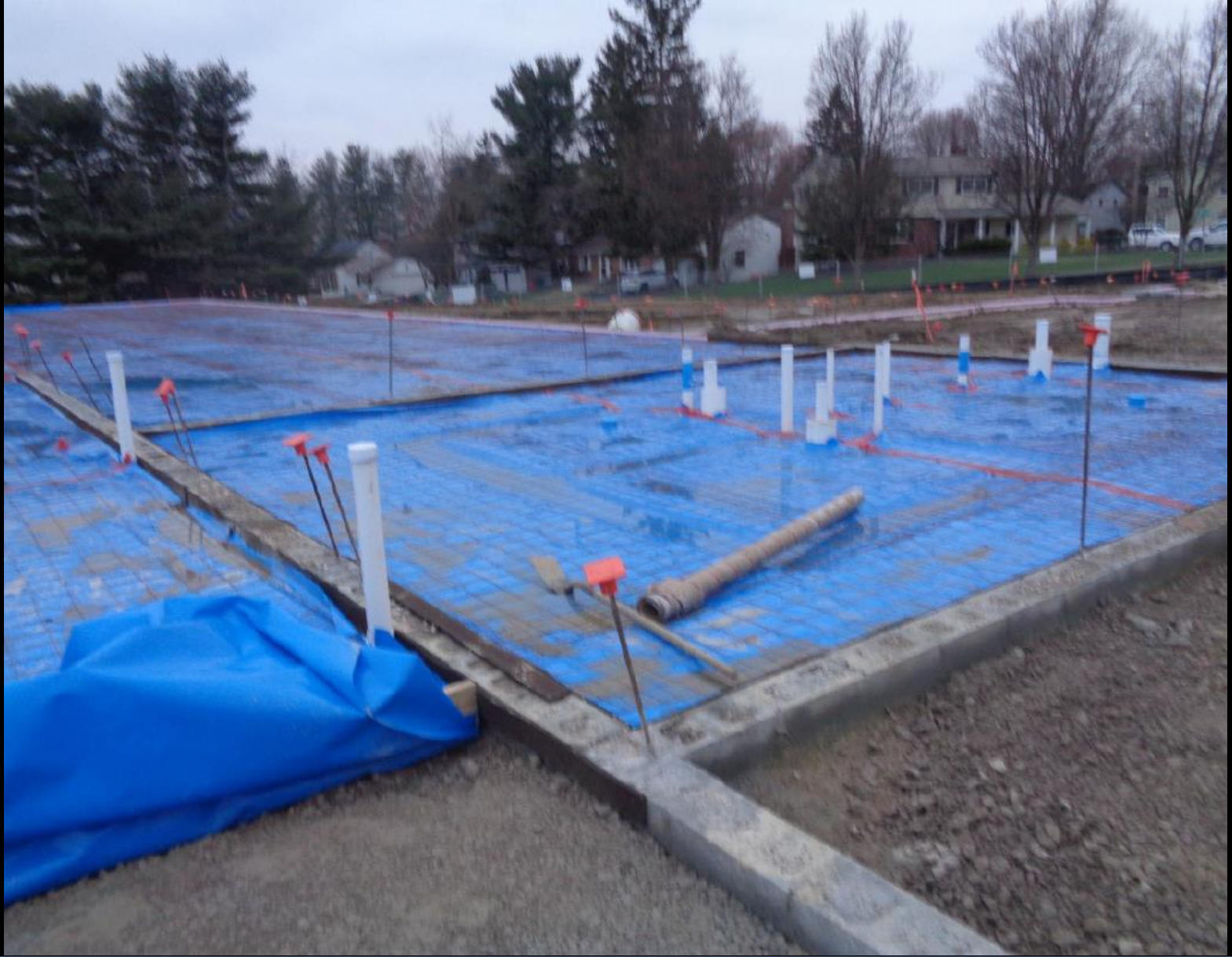
Worthingway Slab Preparation
